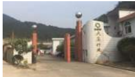
Shunchang Zhujia Bamboo Industrial Co.,Ltd Multi-purpose production facility produces 200,000 m 2 per year.
