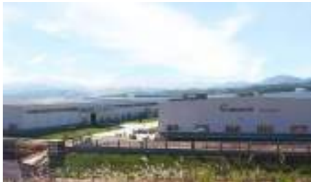
Jiangxi Zhushang Bamboo Industrial Co.,Ltd dassoXTR production facility produces 1 million m 2 per year.
